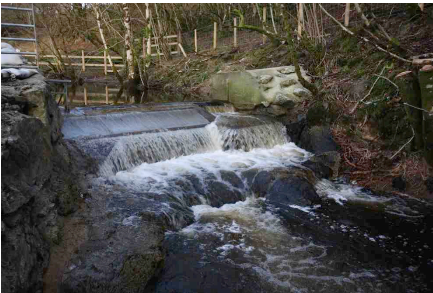
The weir and fish-pass
