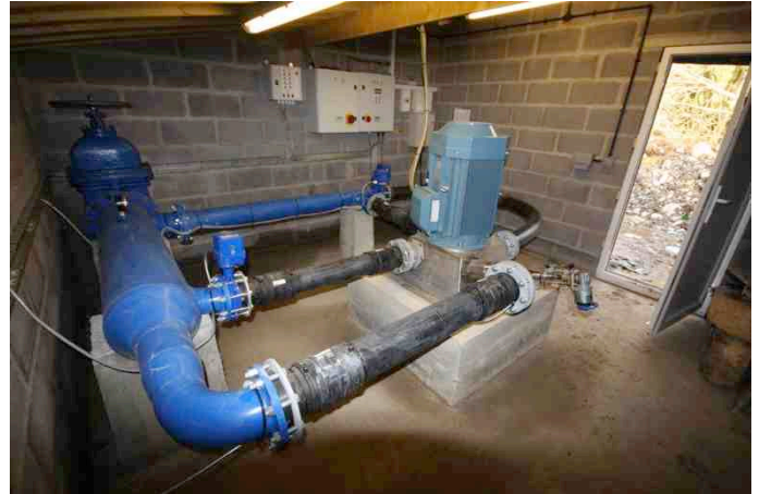
The layout of the Powerhouse
