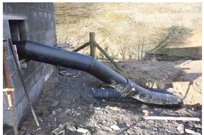
The 'pigging' route and tailrace being installed
